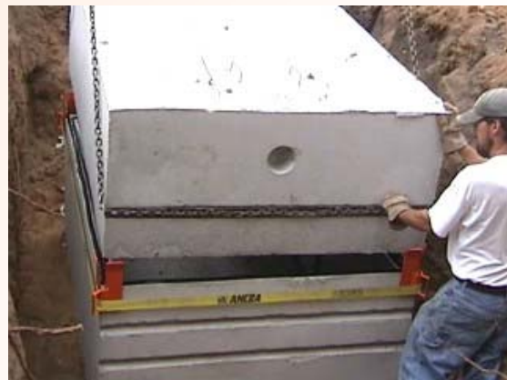
Mid-seam tank installation
